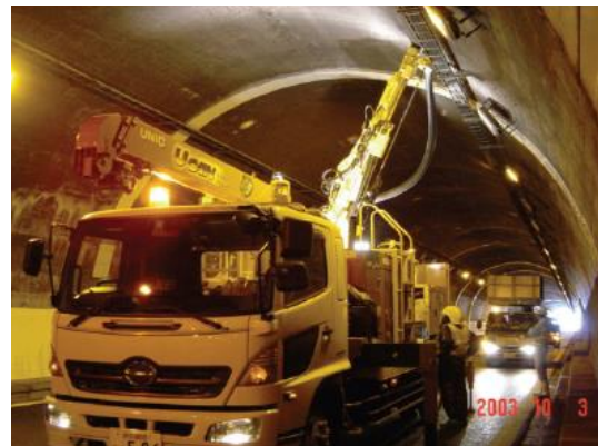
Figure 8. Void detection rotary percussive drilling machine [52]
