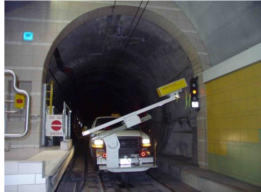
Figure 11. IRIS Hyrail system inspecting a tunnel. Note the capability to be mount on rails [56]
