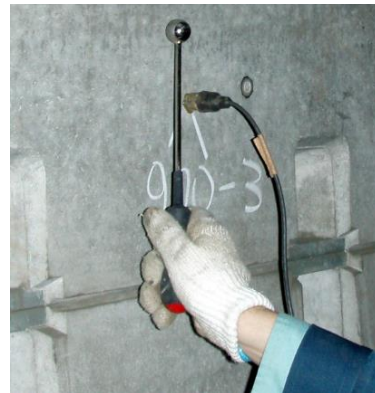
Figure 3. Inspection using an impact hammer [17]
